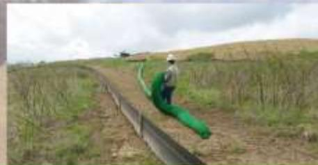
The right choice for removing settleable solids, total suspended solids and turbidity reduction from sediment laden water. Switchgrass Filters are at least as effective as traditional erosion and sediment control BMP's and often are more effective in retaining sediment and other pollutants.
